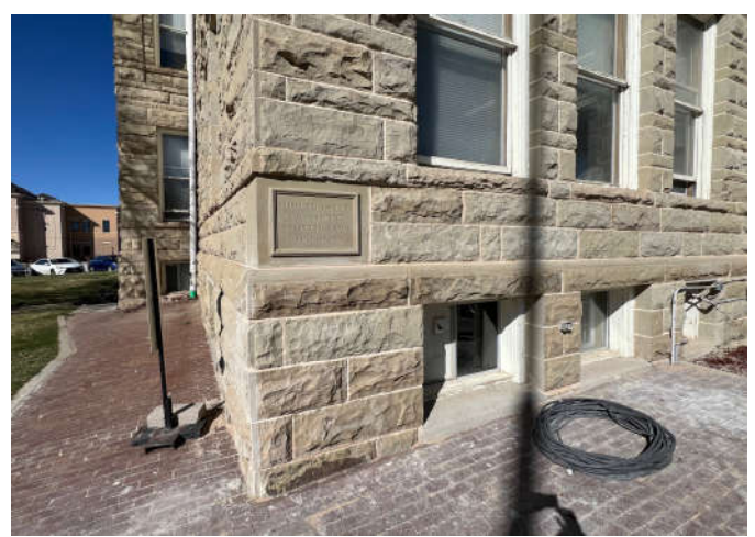
Photo #4: Replacement stone at the bottom of the southeast corner.
