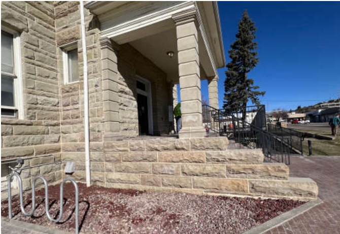
Photo #1: New reconstructed south cheek wall.
