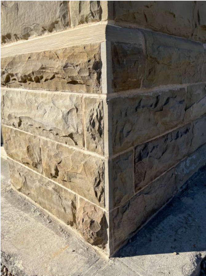
Photo #9: Some tooling remains to be done at the northeast corner.
