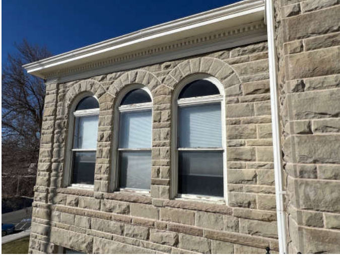
Photo #8: Two holes in the stone located below the frieze were filled.
