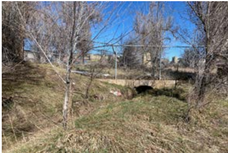
Irrigation ditch on northwest side of property
