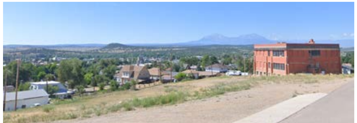
Polk Ave School view from the north, view of adjacent parcel to the east
