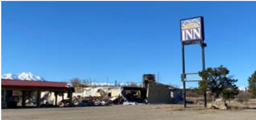
Fire damage on motel and pool house
