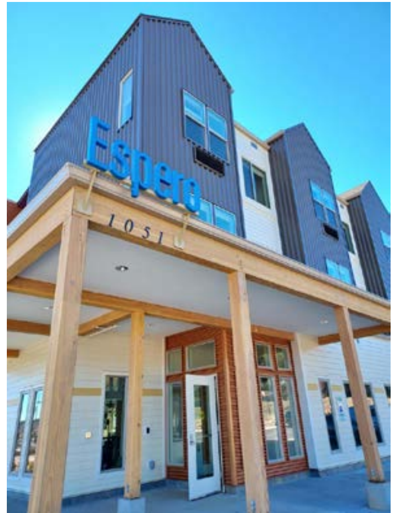
SW Housing Solutions Former Football Field
