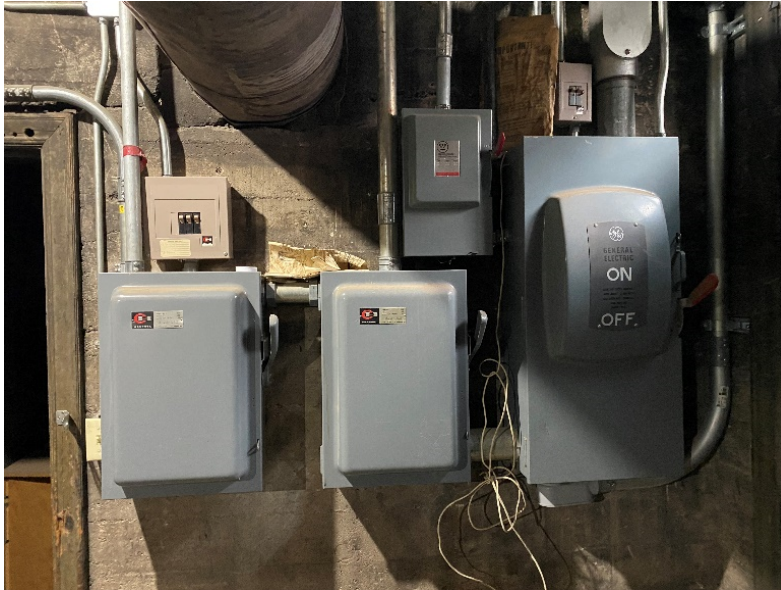
Figure 3: Existing electrical panels, appear older - need to confirm capacity for new use
