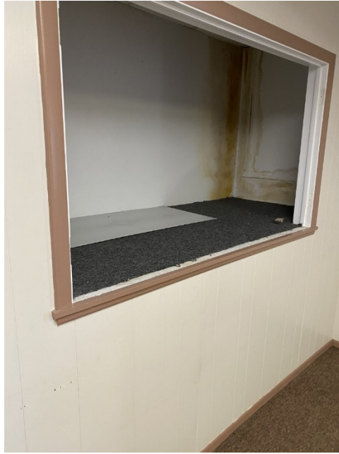
Figure 1: Evidence of water damage
