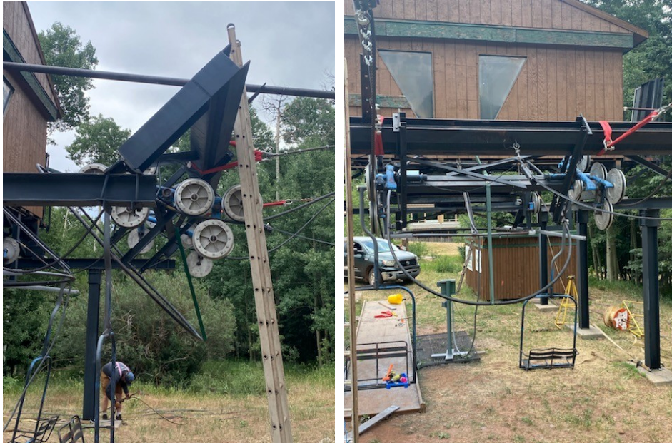
Figure 2 Original incident photos from Panadero staff
