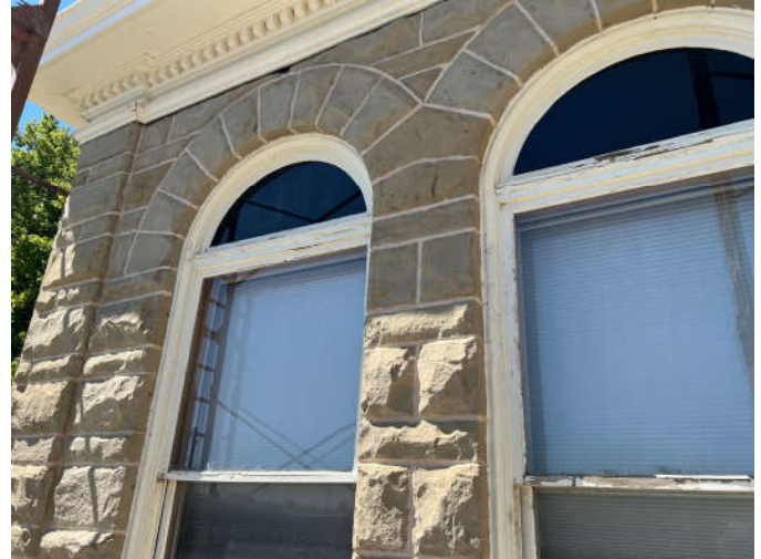
Photo #6: Repointing of the mortar joints is underway, with most joints repointed from the top of the walls to the second floor window sills.
