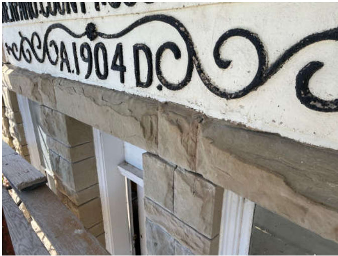
Photo #3: This course of stone, which includes lintels above the window and door openings on the tower's second floor, will be retooled rather than refaced to avoid damage to the plaster sign.
