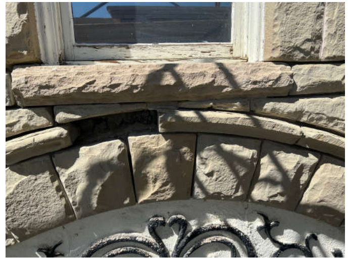
Photo #4: The decorative stone moulding and the small stones below the window sill are eroded. They will be replaced.
