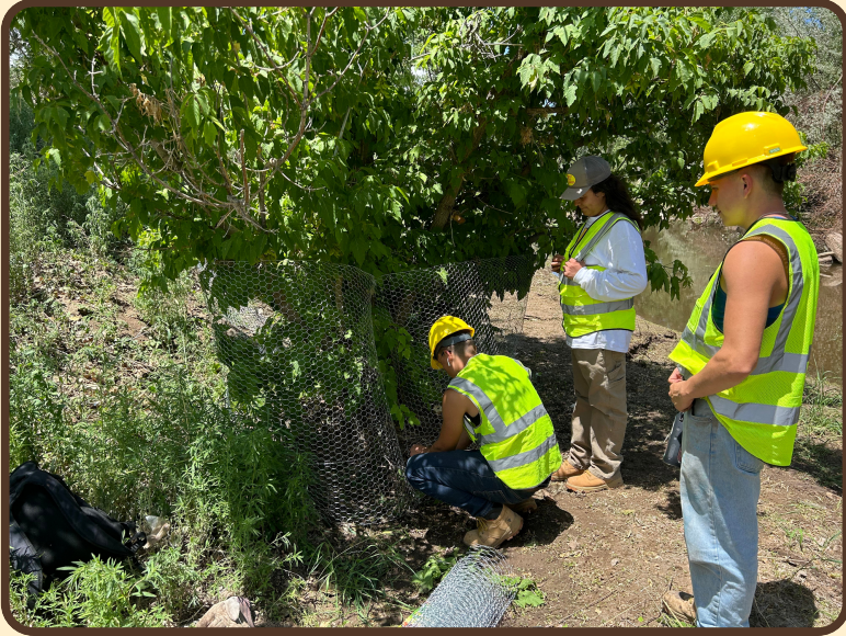
Crewmembers wrapping a couple of bank-side trees
