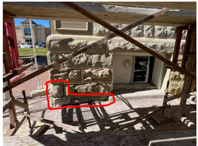
Photo #6: The stones at the bottom of the southeast corner still require replacement. The water table stones above the garden level windows are in poor condition.
