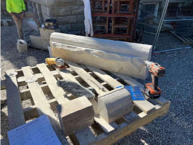
Photo #3: The process for achieving tool marks similar to the original on the radiused top surface of this stone is being tested here.
