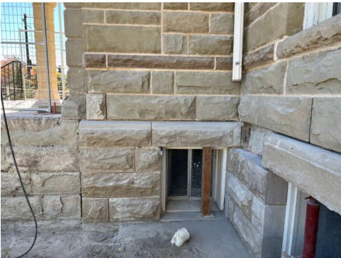
Photo #1: The stones at the bottom of the north tower wall have been replaced. Remaining required effort includes retooling the radiused water table stones and repointing.
