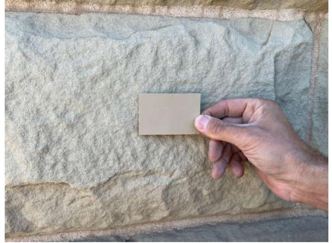
Photo #4: The sheet metal flashing required at the second floor balcony will closely match the color of the stone.
