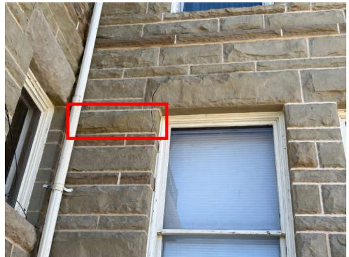
Photo #2: The south bearing stone at this window will receive a deep reface. No pinning is required. However, the lintel stone should be shored prior to refacing.
