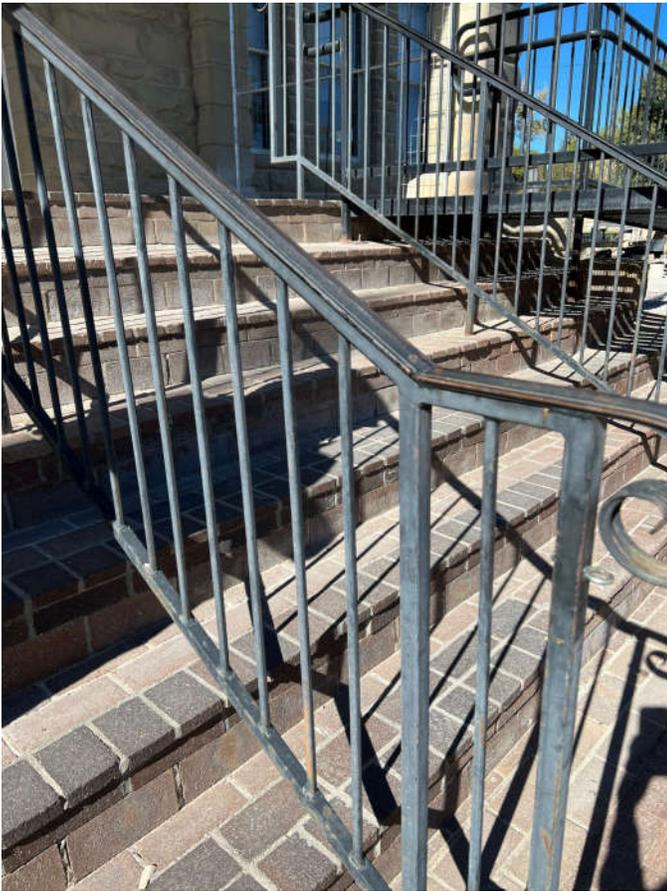
Photo #7: Guardrails are needed along the north and south sides of the main entry porch. Their design should match the existing railing system.
