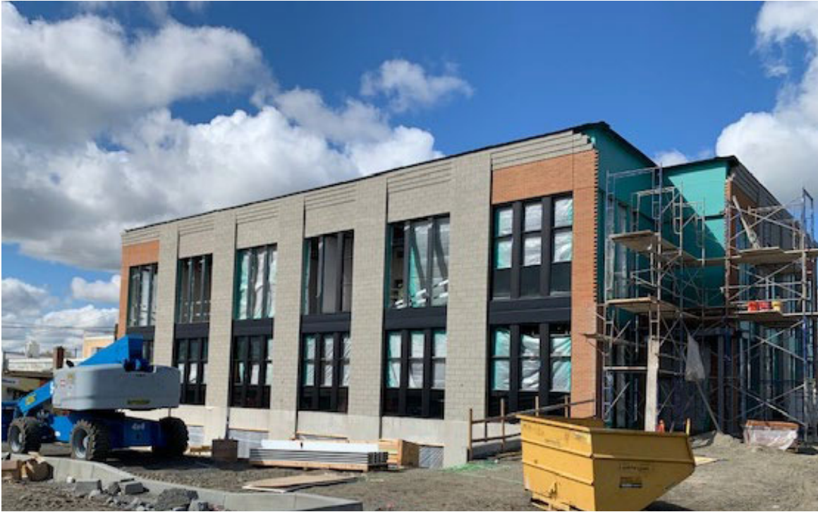
New City Hall Under Construction
