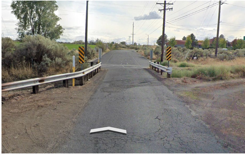
Southbound canal crossing
