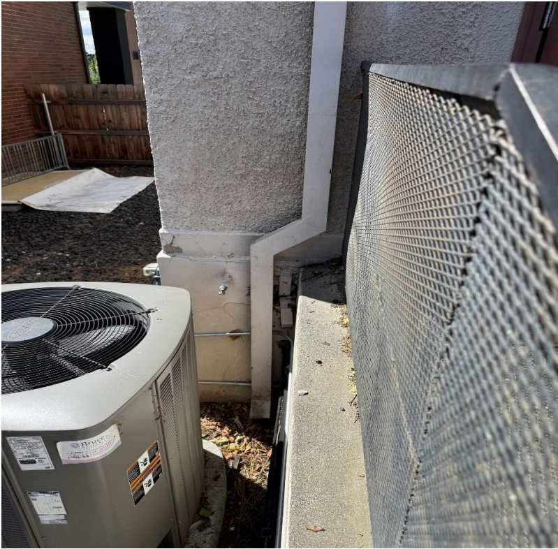
Water damage @ Existing CMU Stem Wall →
