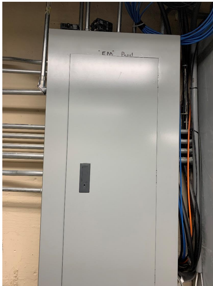
Figure 3 Village Hall Panel EM
