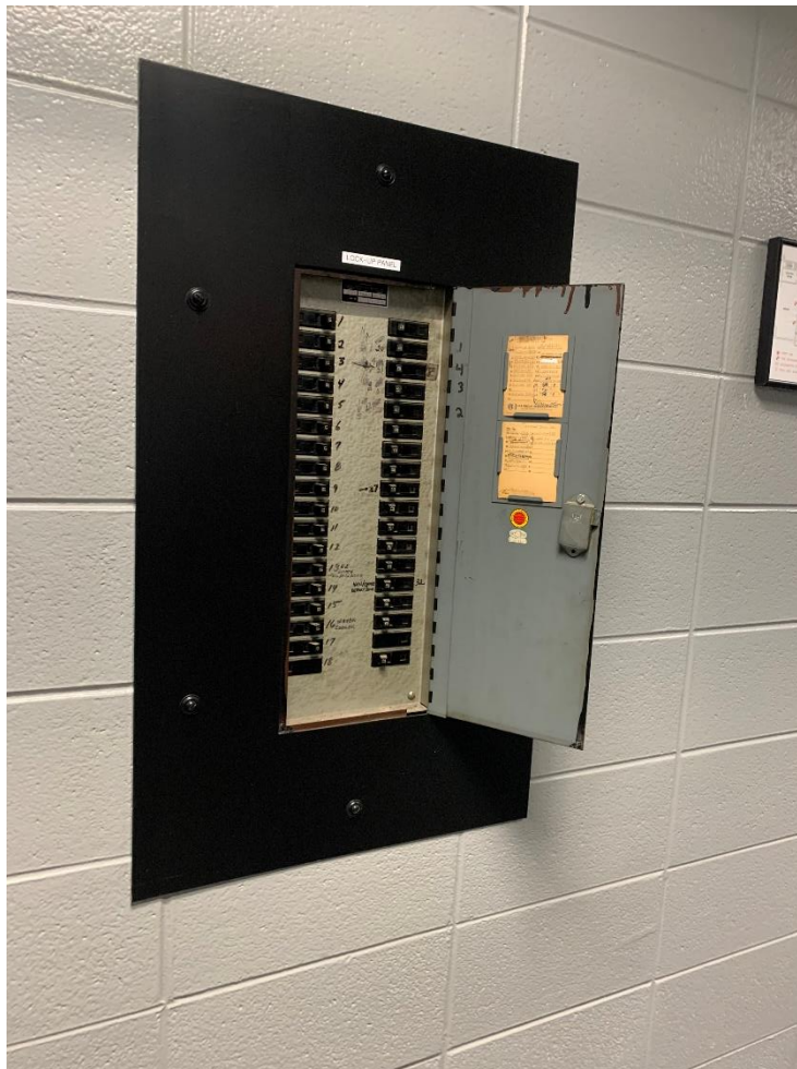
Figure 6 – Police Corridor Power Panel Installation
