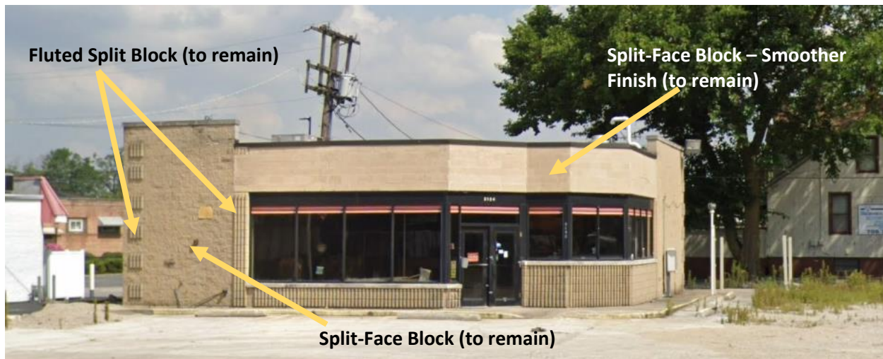
Figure 2: Existing structure on the site with materials identified. Plans for use of materials in redevelopment identified on image.
