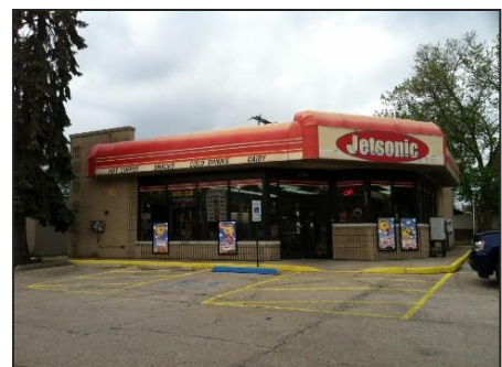
Figure 1: The building's previous use, a Jetsonic convenience store and Citgo gas station, in 2013.
