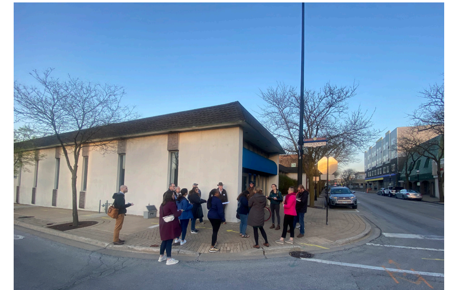
Fig. 23. Site from the Southwest
