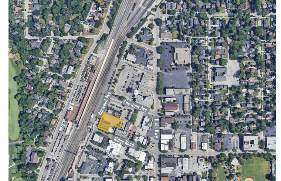
Fig. 22. Aerial View of Site
