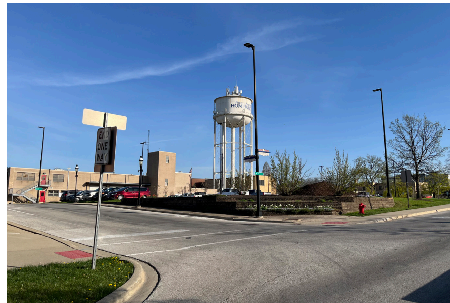
Fig. 21. Site from the Northwest
