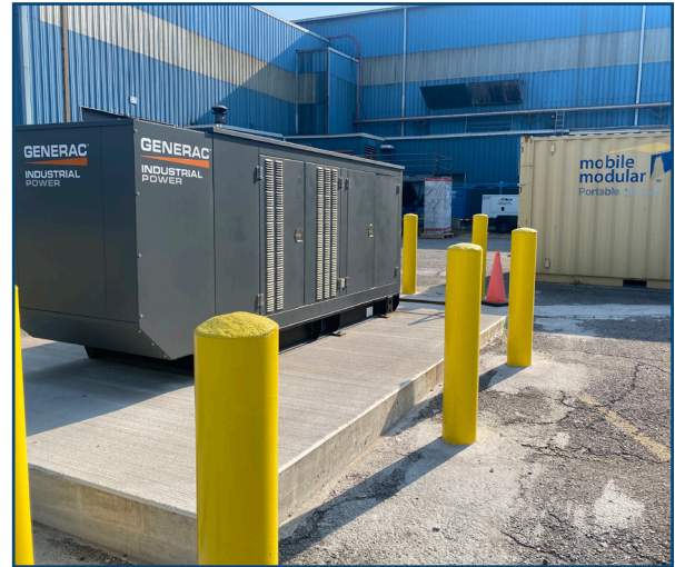
New Backup Electrical Generator Installed for NMLK Indiana
