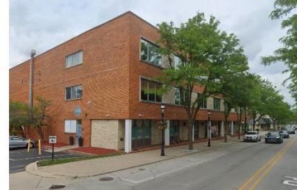
Figure 1: Golden Eagle Office Center in 2025
