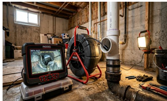
Televising a Sewer Cleanout
