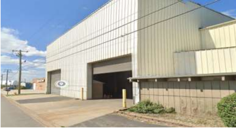
1510 175 th St. (west of the Project Site on the north side of 175 th St.)
