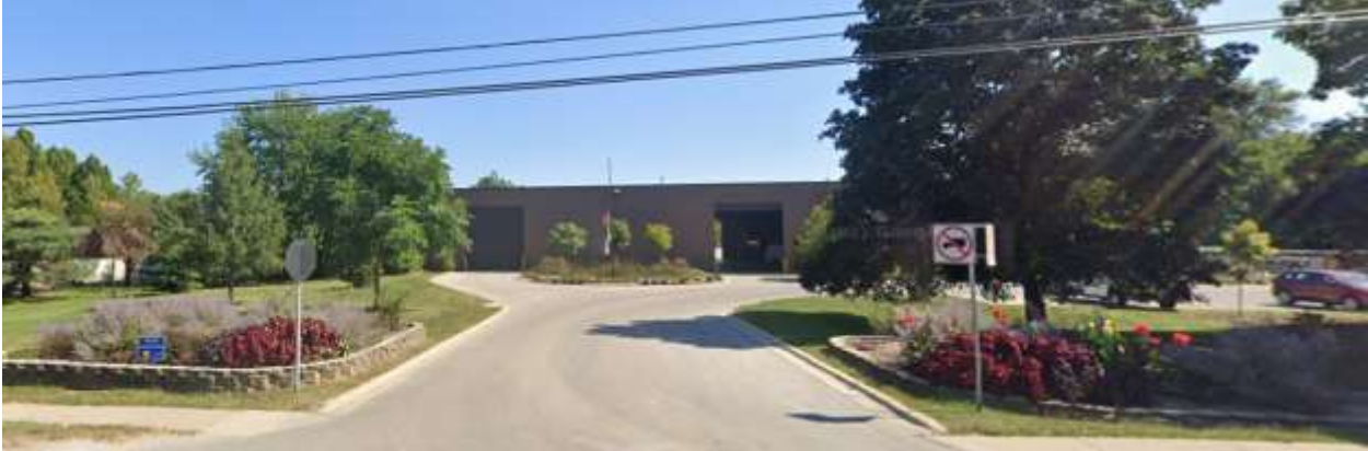
17768 Ashland Ave., Homewood, Illinois
