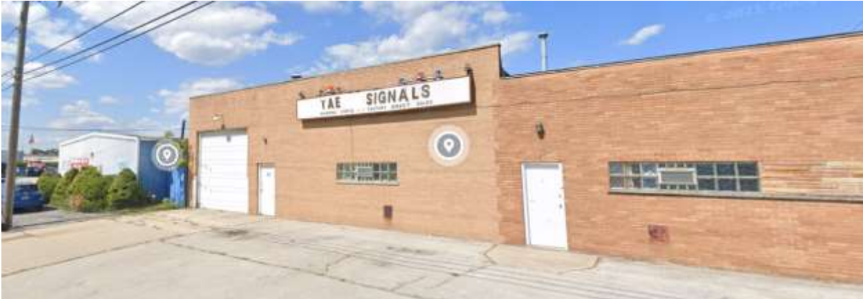
T.A.E. Signal located at 1516 175 th St. (west of the Project Site on the north side of 175 th St.)
