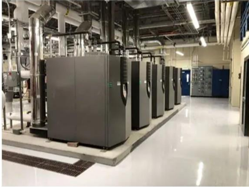
High-efficiency boilers
