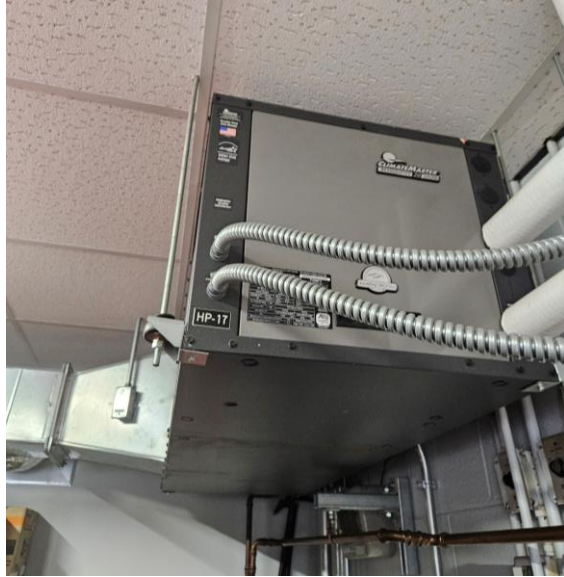
Typical ducted ground source heat pump
