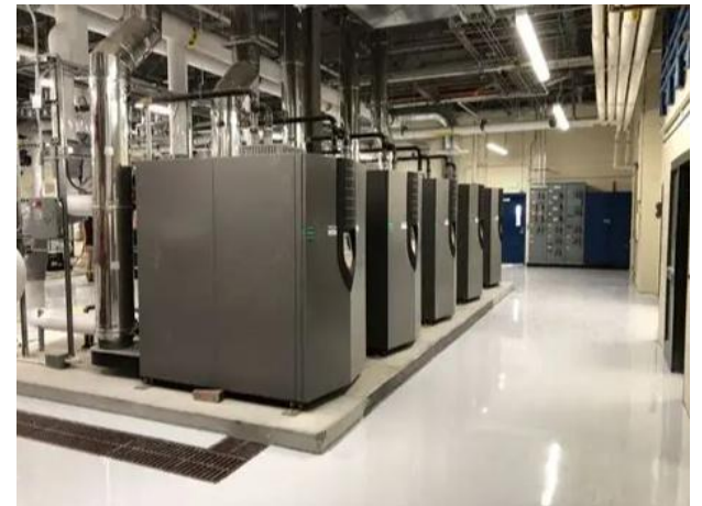
High-efficiency boilers
