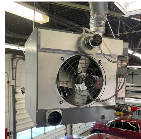
Typical gas-fired unit heater
