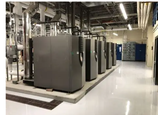
High-efficiency boilers
