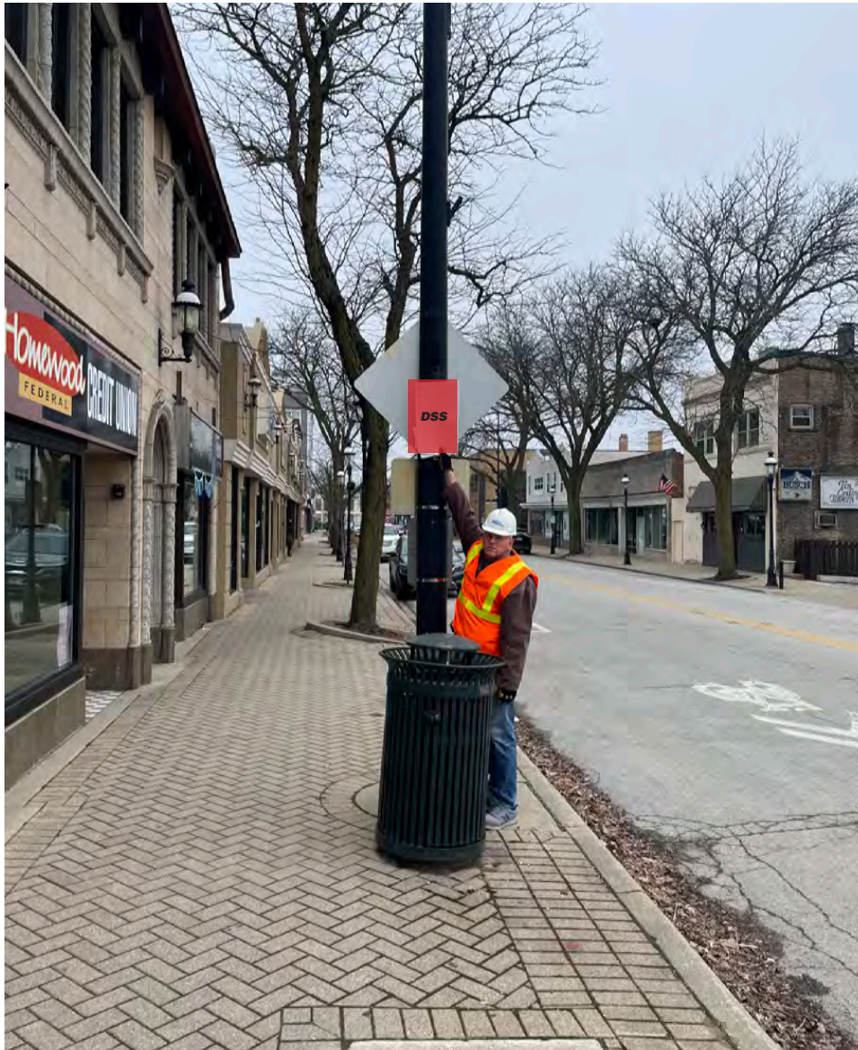
New sign panel mounts to existing lamp post, banded above HM1-045-W.
