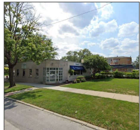
Figure 1: Existing Building @ 18114 Gottschalk Avenue (2025)
