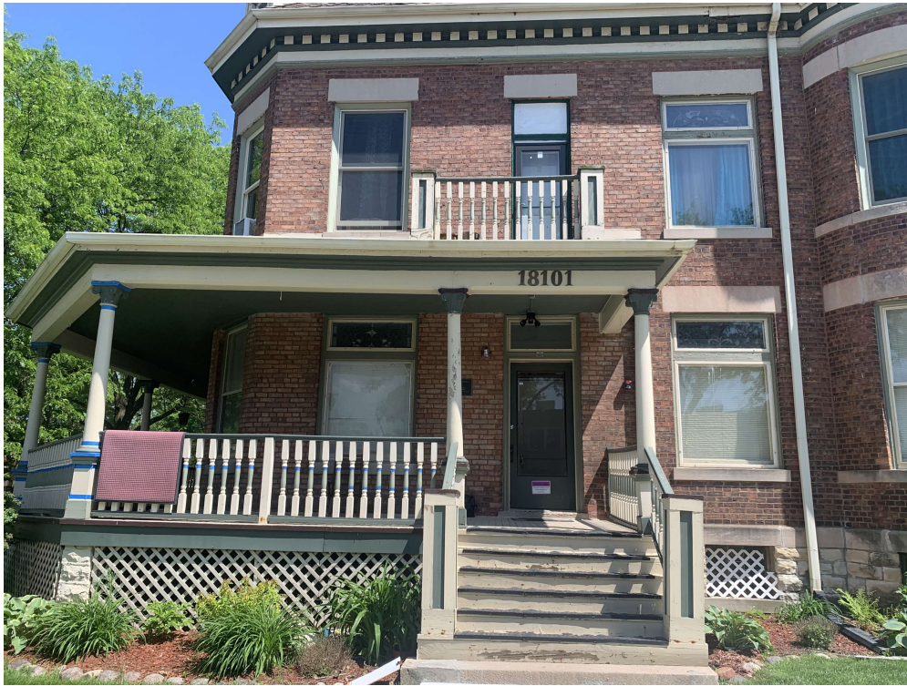
STREET VIEW OF FRONT PORCH
