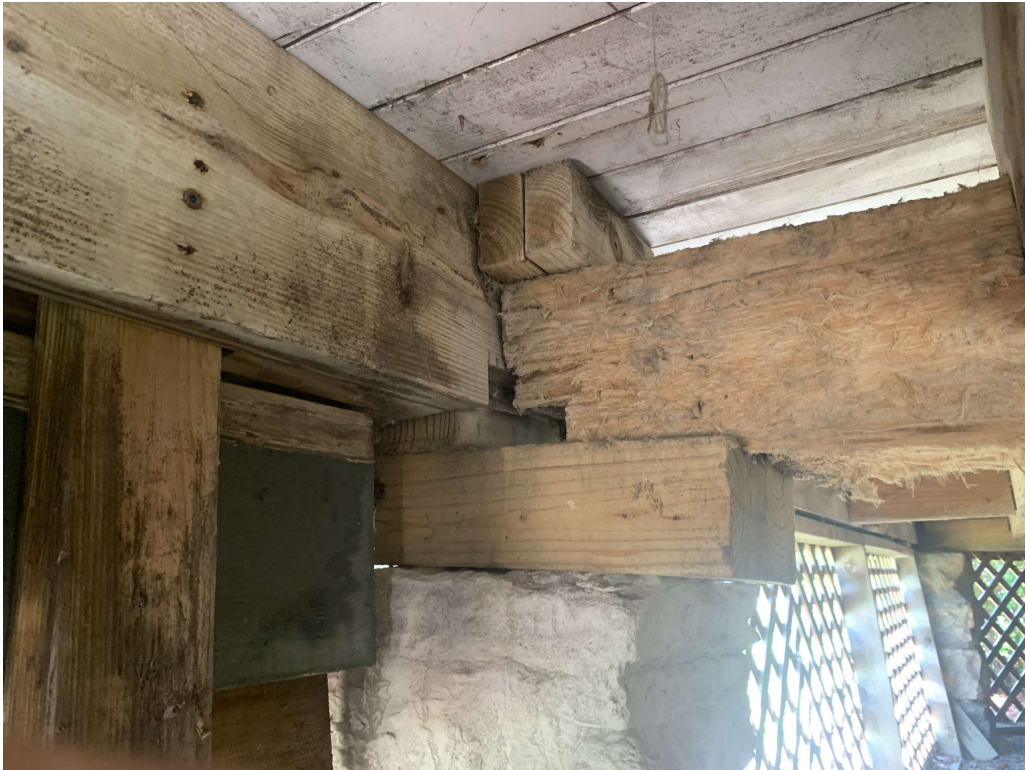
BEAM ON STONE PEDESTAL & BLOCKING
