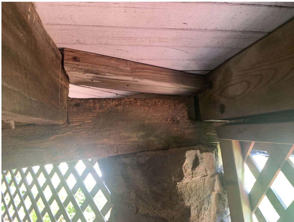
BEAM ON STONE PEDESTAL & BLOCKING
