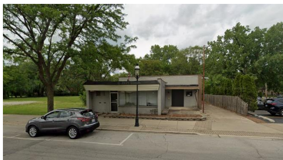
Figure 2: The subject property photographed in July 2025 (Source: Google Maps, 2025 imagery)
