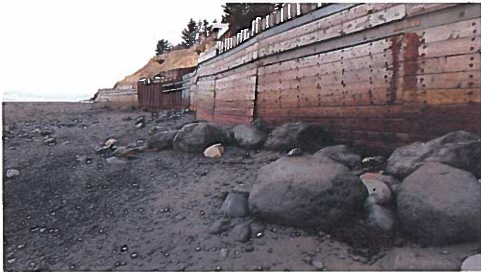
Figure 2 - January 2019 East Portion of Wall
