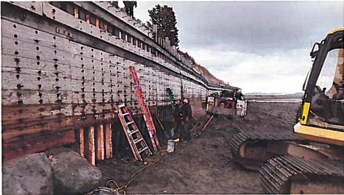
Figure 1 - January 2019, replacing vertical posts to allow installation of new horizontal timbers.
