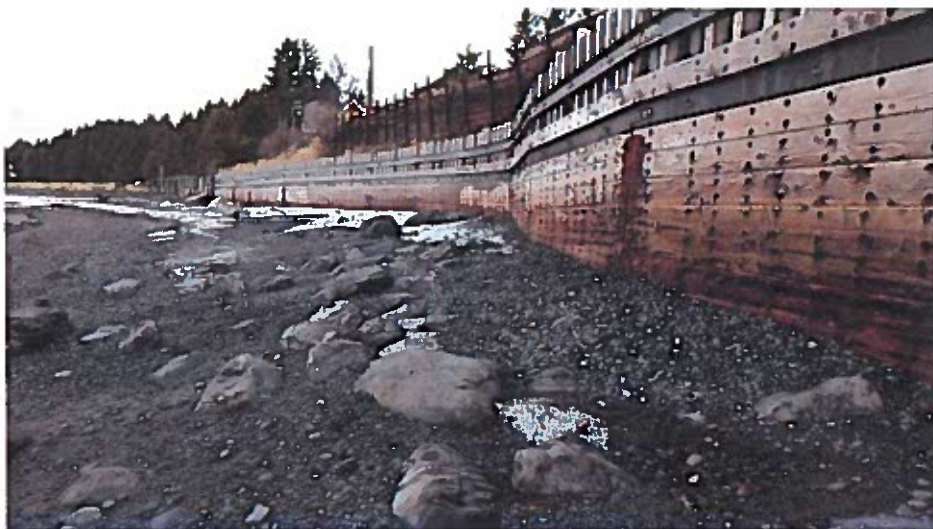
Figure 3- January 2019 West Portion of Wall
