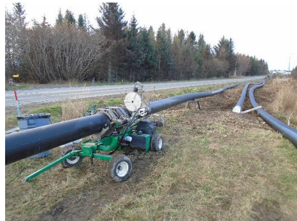
40' long, 12" HDPE water main sections being "fused" together in preparation for installation along Kachemak Drive
