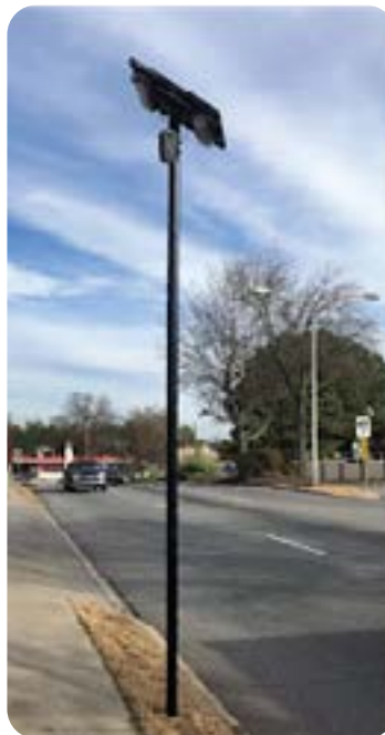
Entrance to Hotel Solar & Flock 14 foot pole
