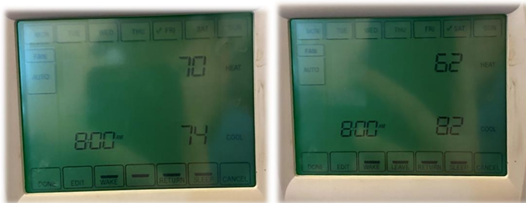
Figure 8. HVAC operation setpoints for the occupied week-day schedule (left), Setback setpoints for the unoccupied week-end schedule (right).
