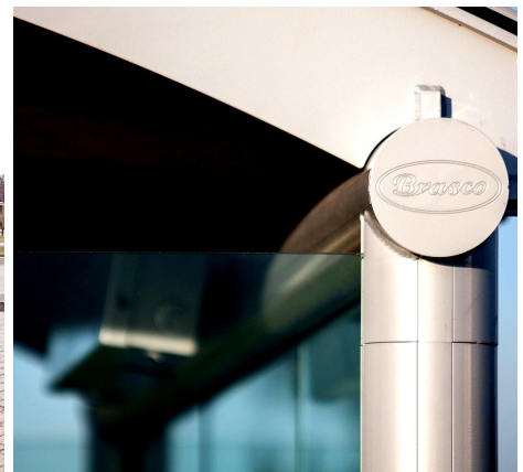
Eclipse Header and Side Wall Demonstrating Concealed Fasteners and Pocketed Columns
