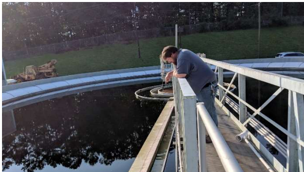
A utility mechanic inspects a mechanical arm on the Wastewater Treatment Plant's clarification tank, which sweeps the water surface of large organics and trash.
