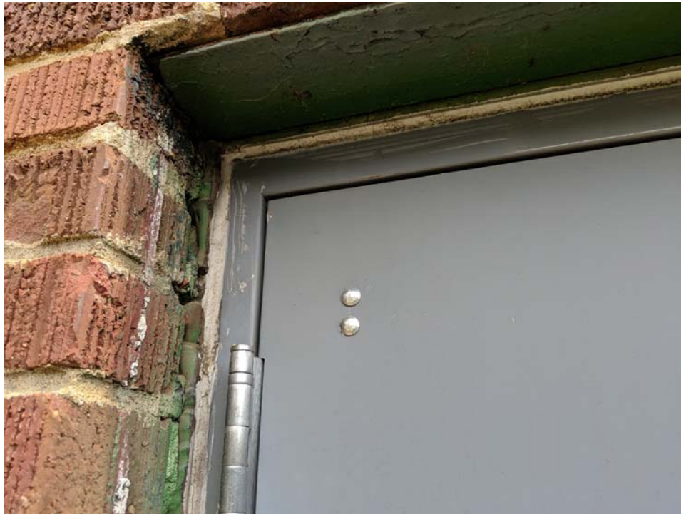
Door caulk on original brick structure.
