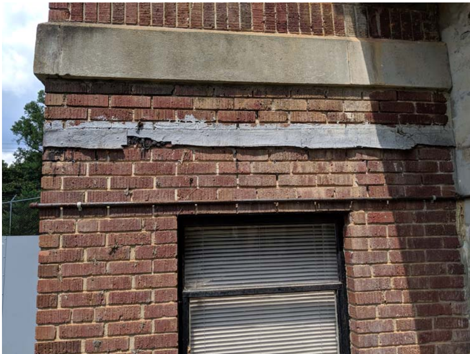
Asbestos containing flashing on C Side.
