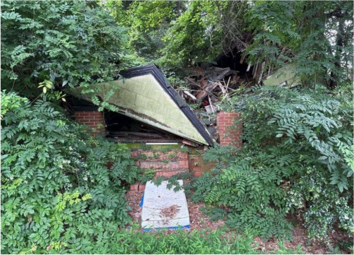
Junk Accumulation(s)- 370 Cornelius Street
