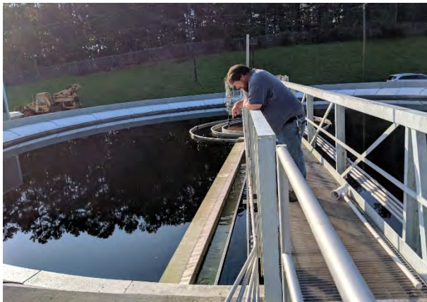
A utility mechanic inspects a mechanical arm on the Wastewater Treatment Plant's clarification tank, which sweeps the water surface of large organics and trash.
