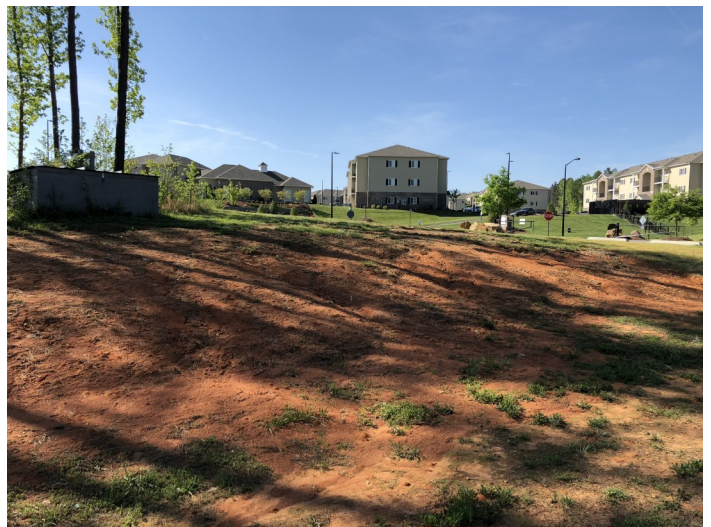
Eroding slope beside multi-use field
