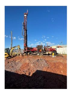
Cluff drilling continues to drill Replacement Well 17. They are at 300 feet deep with about 200 – 400 feet remaining.
