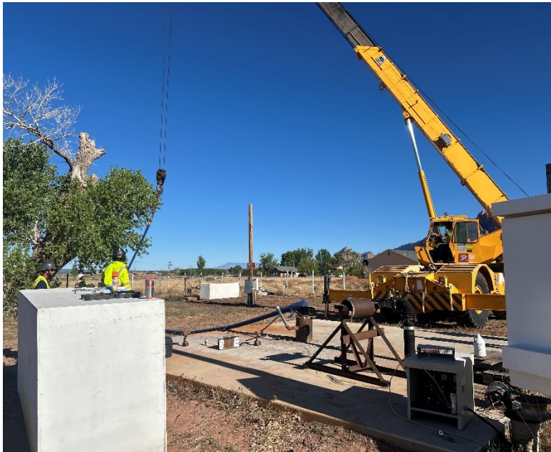
(Crew Pulling the Pump and Motor)
