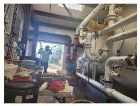
The filters were, cleaned, sanitized, and returned to service. Mayor Allred, Vance and Eric visited the water-plant to see the progress there. I have a quote to replace the media in the east side. The east side filters have a sand based media that we would like to replace with this mineral based media which appears to be a high grade longer lasting media.
