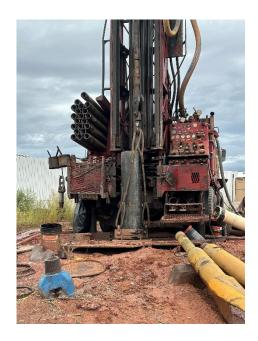
Cluff drilling continues to drill replacement Well 17 and have installed casing to the depth of 560 feet. To date the well has been drilled to over 600 feet in depth.
