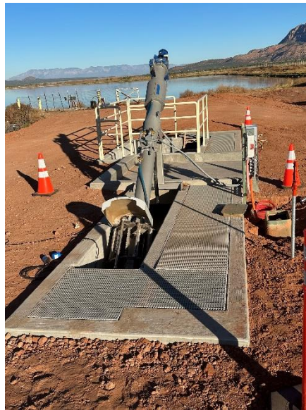
(Headworks Building & Headworks Screen)
