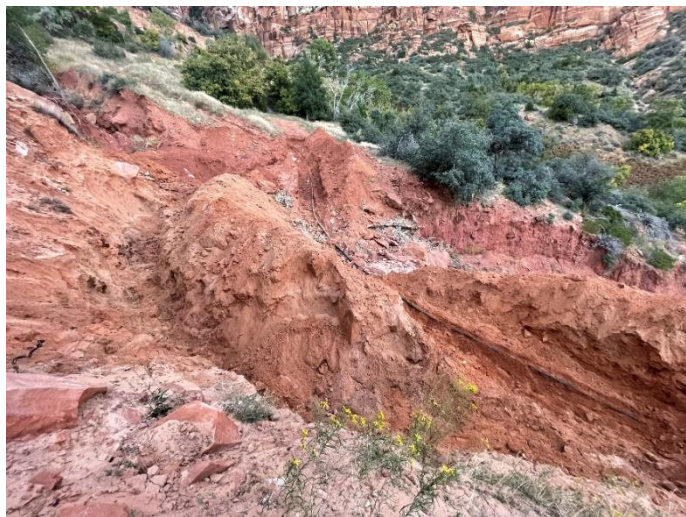
(Maxwell Canyon Line Repair)
