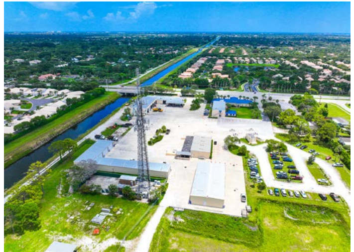
[LWDD Headquarters, Delray Beach, FL]
