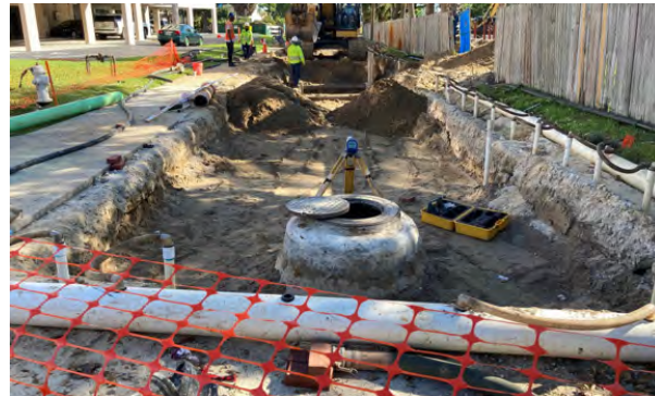
Clemons and Saturn St. Stormwater and Sewer Improvements
