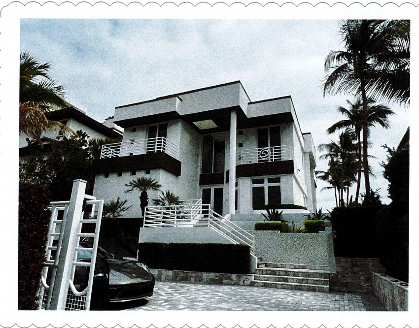
3 EXISTING CONDITIONS (FRONT) N.T.S.
