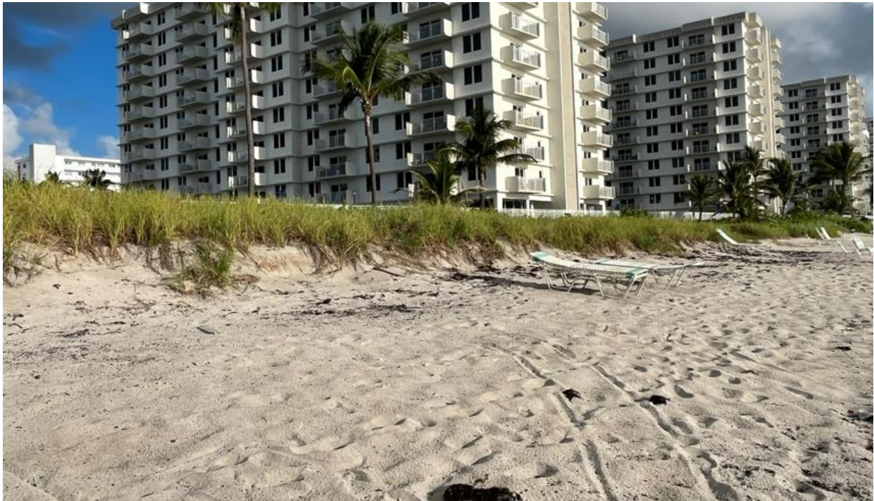
Photo 7. View to the north along the beach in front of the Ambassadors South Condo. Note the scarped dune face and dune toe.
