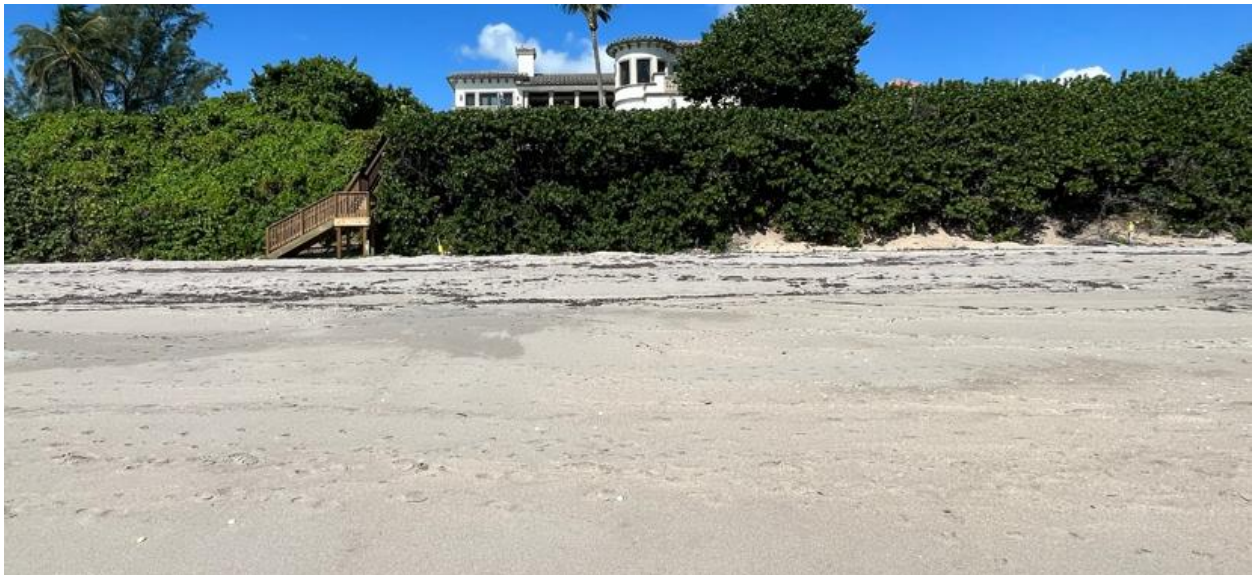
Photo 12. Some properties to the north of Yamato Rock have densely vegetated, high dunes; however, undermining is occurring at the base of these plants, with ~4-5 feet of scarp in some areas north of the stairs.
