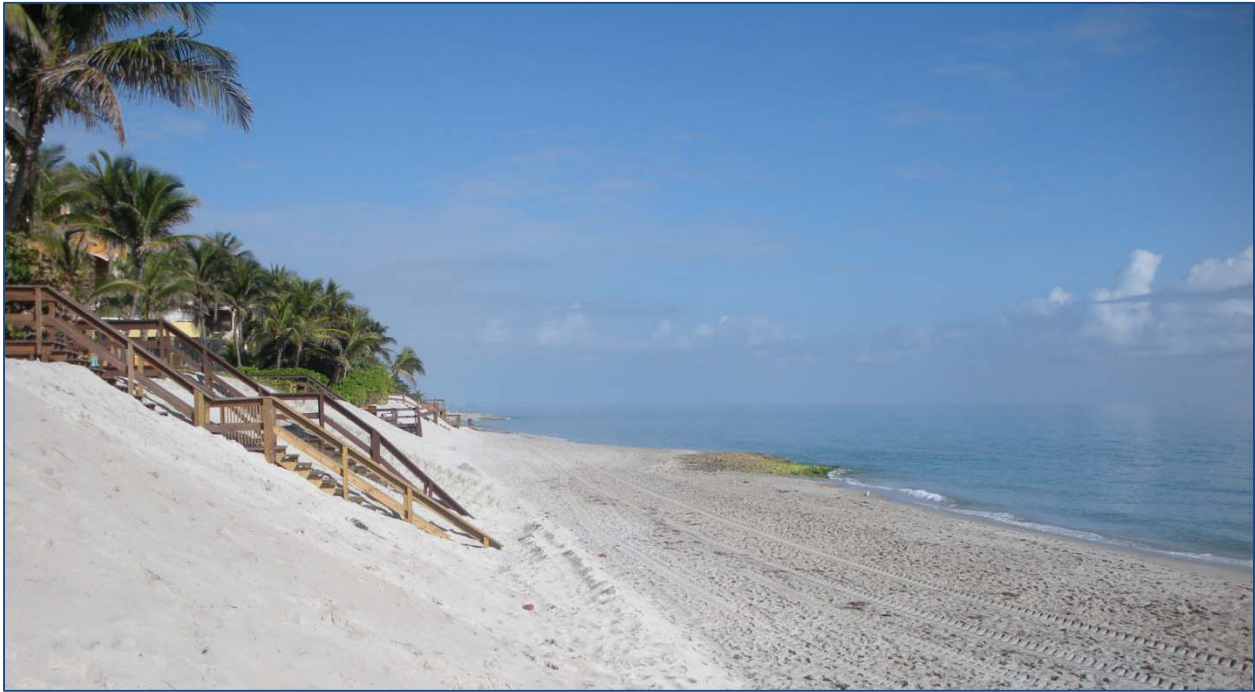
Photo 5. View Looking north from the Ambassadors Condominium. Note the rock outcrop and newly rebuilt dune in front of Ocean Place Estates.
