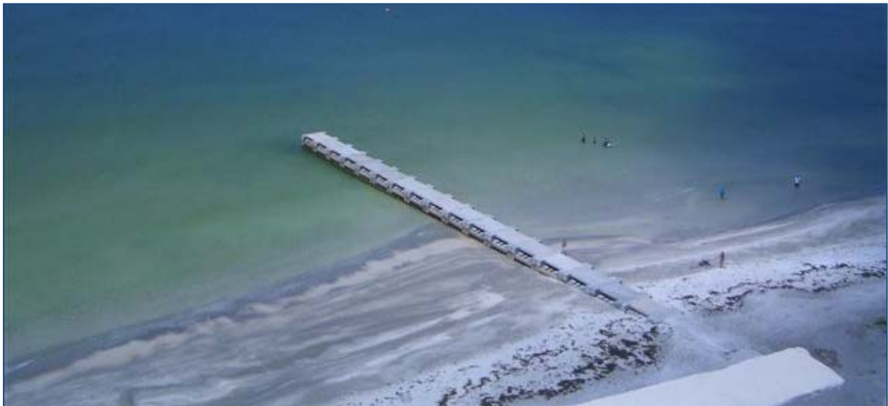
Photo 10. Permeable adjustable groin in Longboat Key. Note the shoreline offset on the left (south) side of the groin compared to the right (north) side of the groin.
