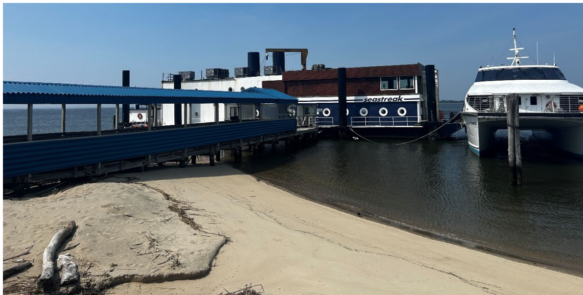
Seastreak ferry terminal.
