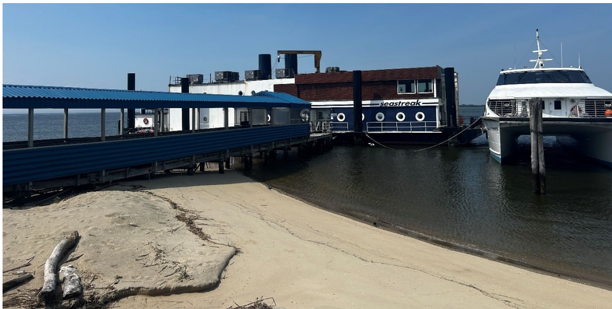
Seastreak ferry terminal.
