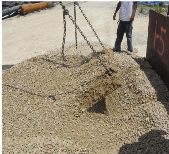
Figure D-4. The steel plates are tilted to facilitate exhumation.
