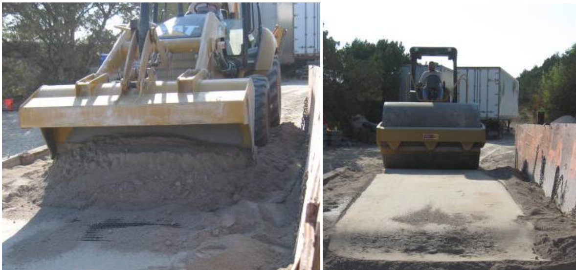
Figure D-2. Grid positioned over compacted base and covered. Cover soil/aggregate is uniformly spread and compacted using field-scale equipment and procedures.
