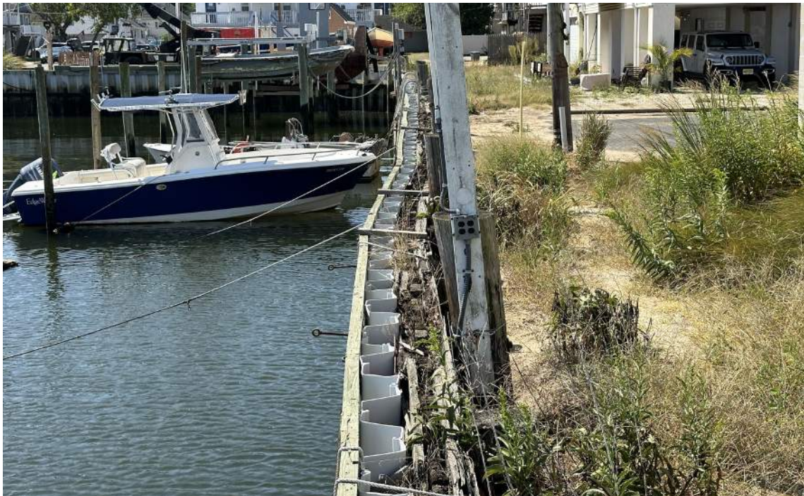
Photo 32: Section C , Westerly Bulkhead, Bulkhead Line, View 2
