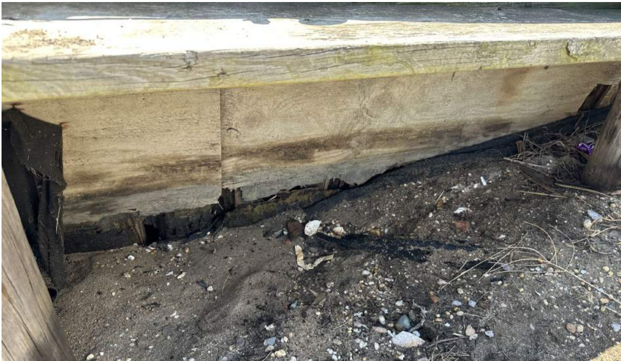
Photo 28: Section C , Westerly Bulkhead, Plywood backing Steel Sheet Piles, View 1
