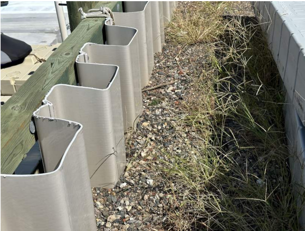
Photo 8: Section A, Easternly Bulkhead, View 2
