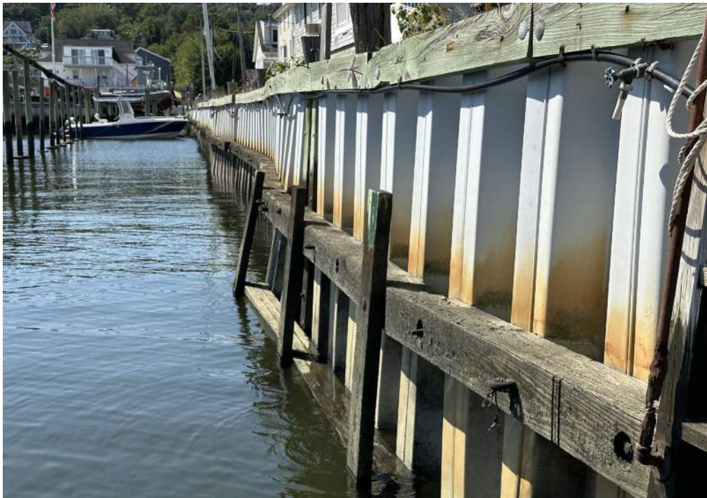
Photo 36: Section C , Westerly Bulkhead, Bowed Out Bulkhead Repair, View 3
