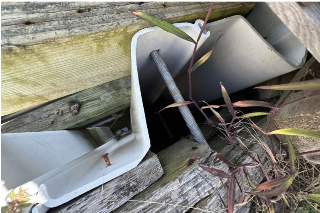
Photo 19: Section B , Southernly Bulkhead, Vinyl Bulkhead Connection
