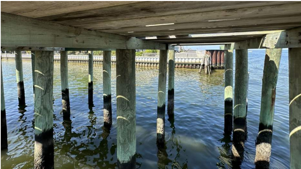
Photo 41: Section D, Easternly Dock, Girder to Pile Connection, View 2
