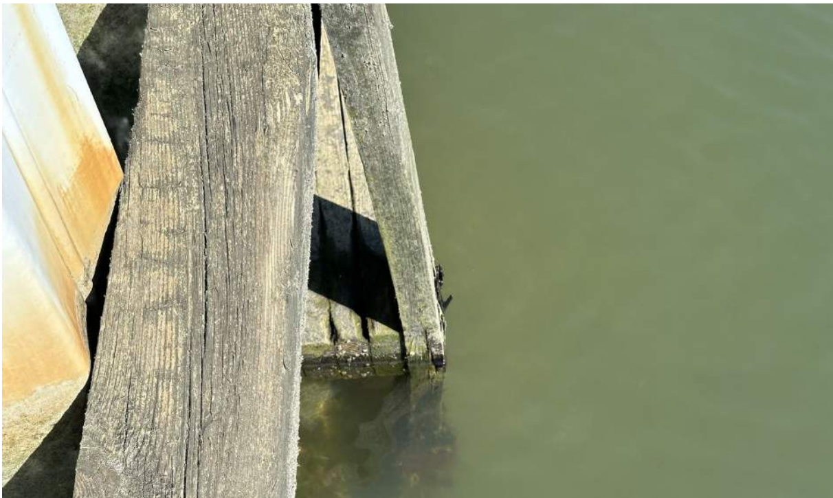
Photo 35: Section C , Westerly Bulkhead, Bowed Out Bulkhead Repair, View 2
