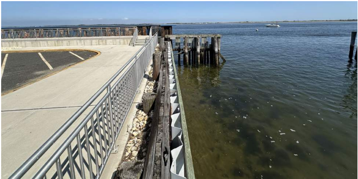
Photo 38: Section C, Westerly Bulkhead, Bulkhead Along Marine PI
