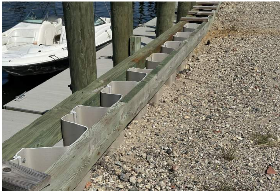
Photo 2: Section A , Easternly Bulkhead, Viewed from Grade
