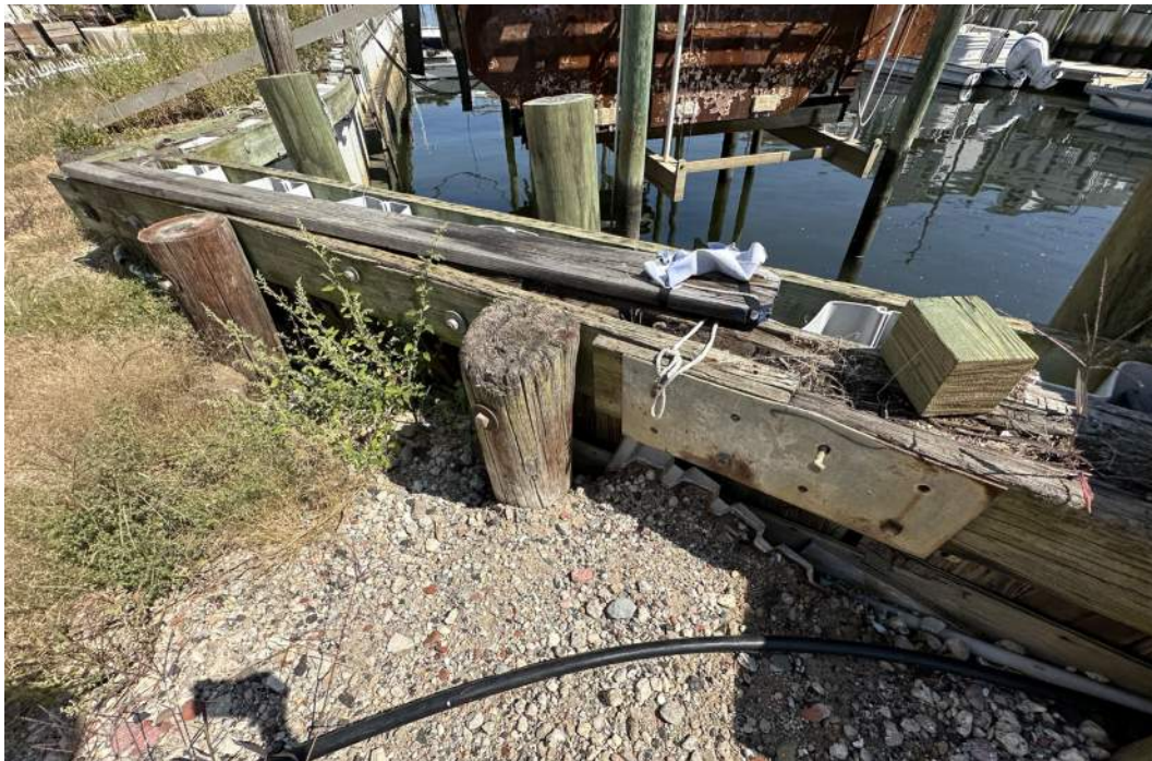
Photo 16: Section B , Southernly Bulkhead, Corner with Westerly Bulkhead, View 2
