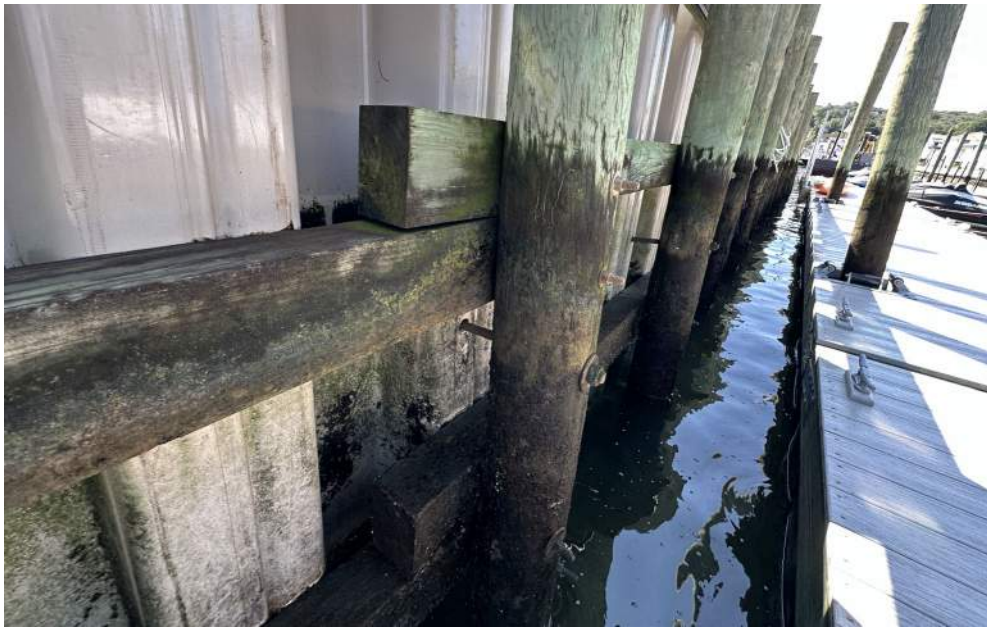
Photo 6: Section A, Easternly Bulkhead Water Lap Connection, View 2
