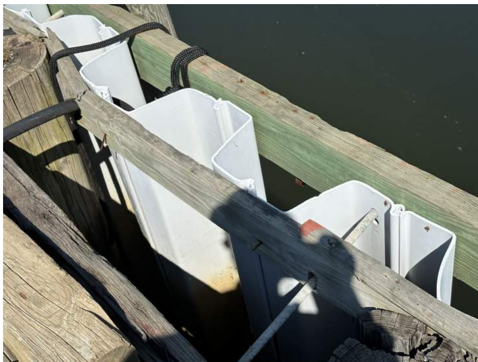
Photo 13: Section B , Southernly Bulkhead, Viewed on Angle from Grade, View 1
