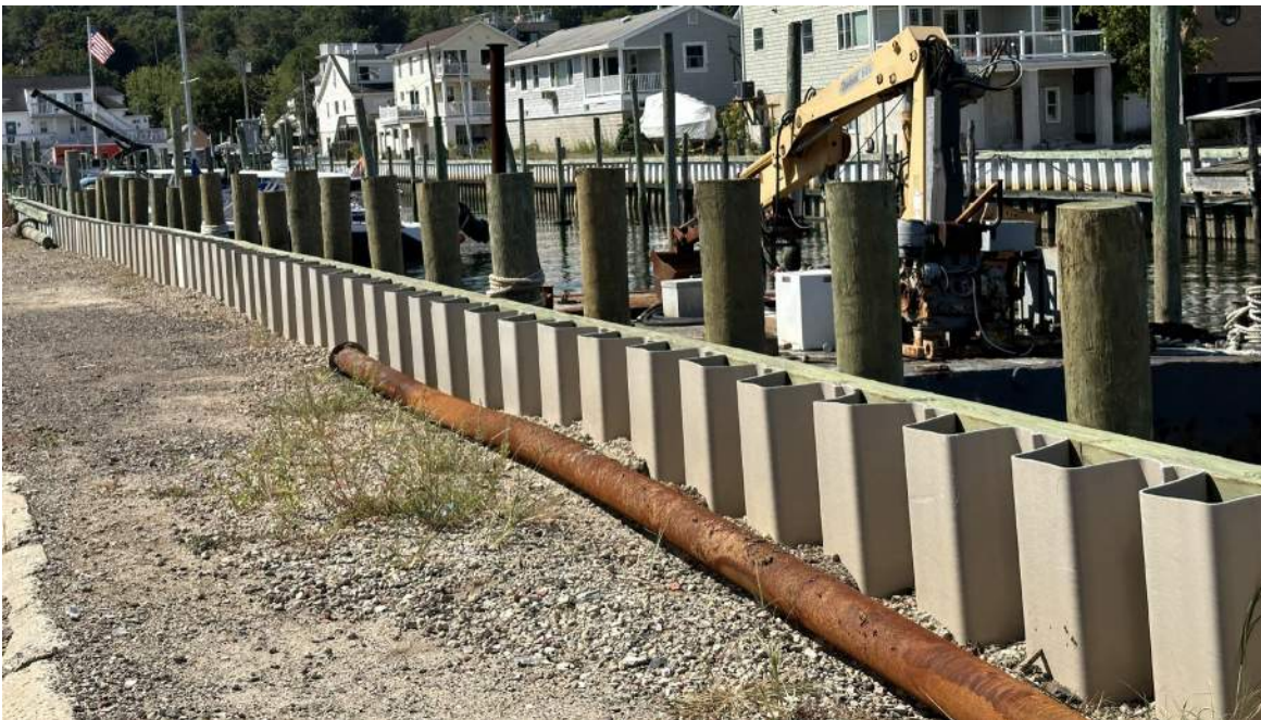
Photo 7: Section A, Easternly Bulkhead, View 1
