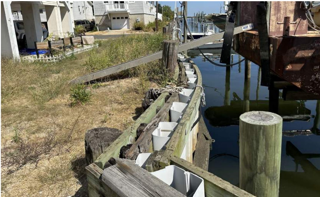
Photo 21: Section C, Westerly Bulkhead, View from grade
