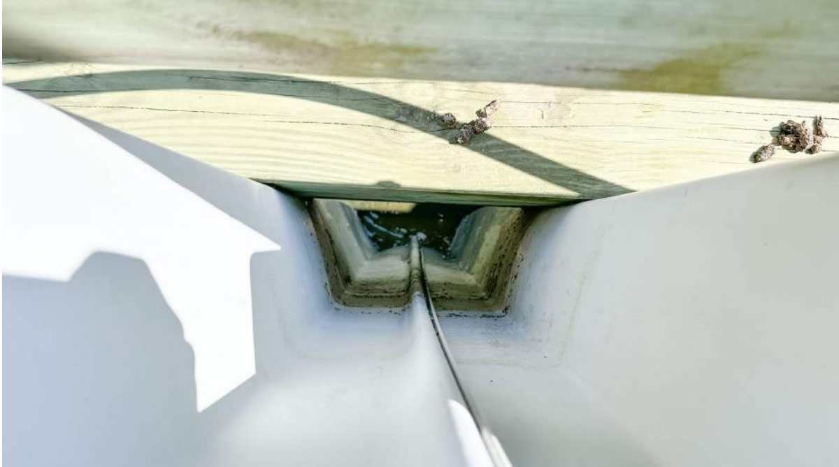
Photo 20: Section B, Southernly Bulkhead, Viewed down Sheet Pile
