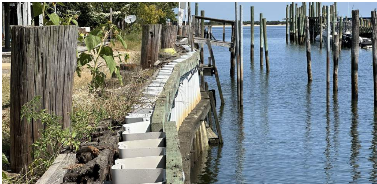
Photo 33: Section C , Westerly Bulkhead, Bowed Out Bulkhead Repair
