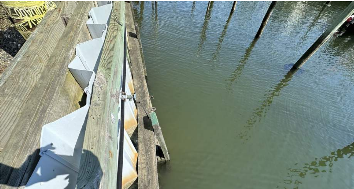
Photo 34: Section C , Westerly Bulkhead, Bowed Out Bulkhead Repair, View 1
