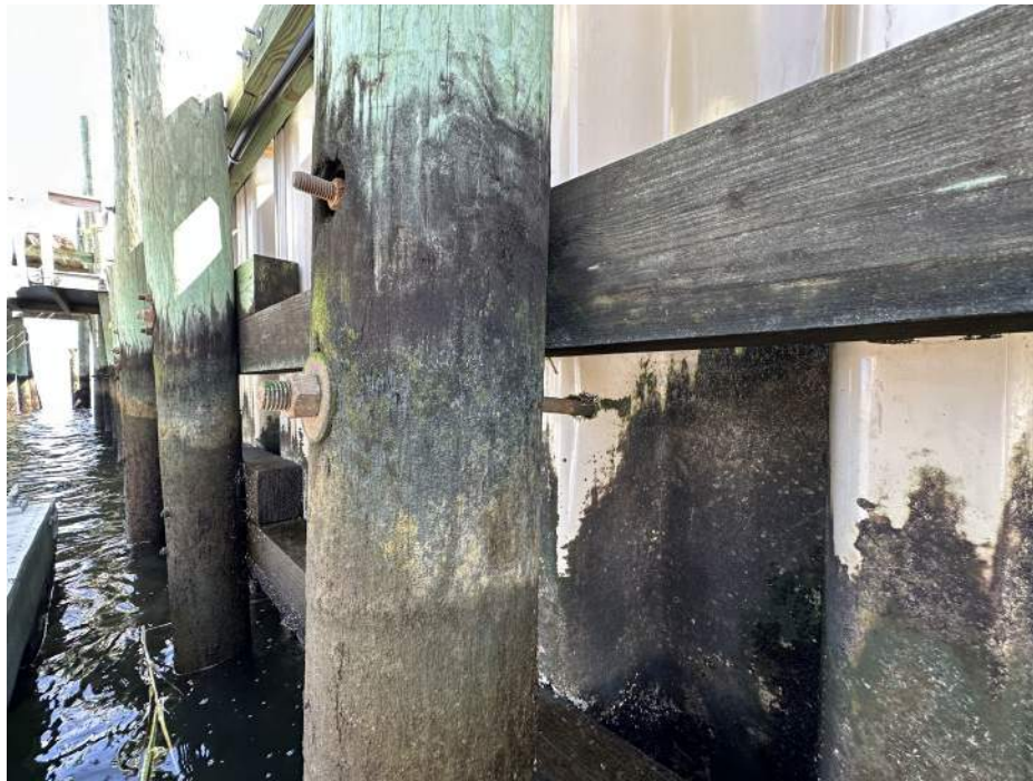
Photo 4: Section A, Easternly Bulkhead Exposed Fastening System View 2
