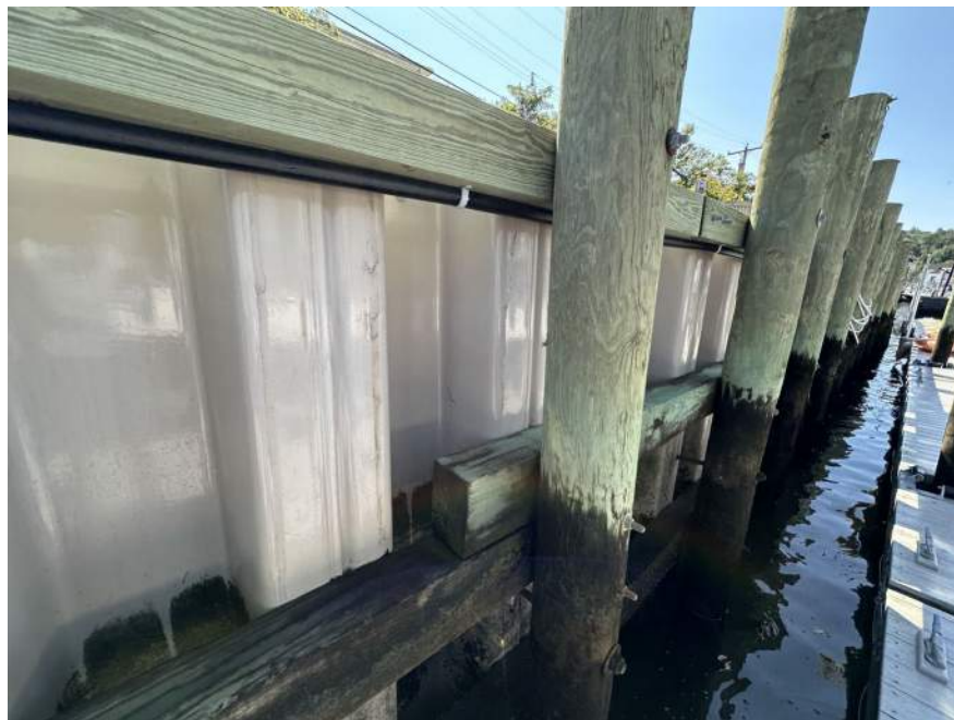
Photo 3: Section A , Eastern Bulkhead Piles, Sheet Piles and Walers Viewed from Floating Dock Infront of Bulkhead
