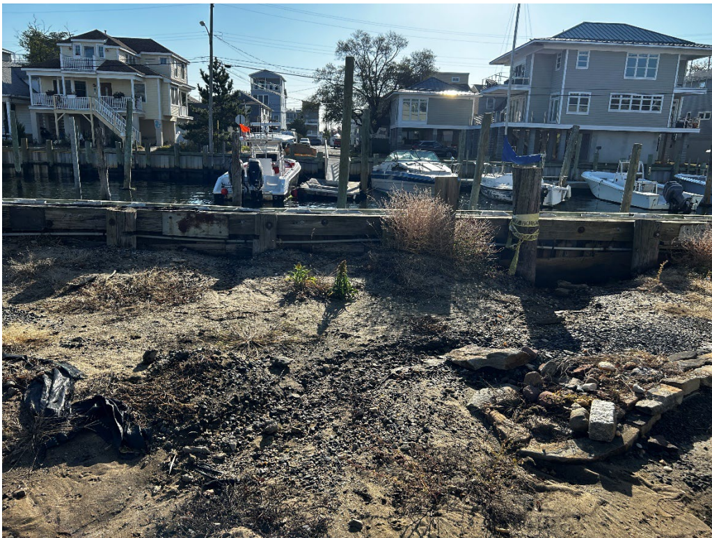
Photo of the Westerly Bulkhead (10-21-2024)(Provided by HGA)
