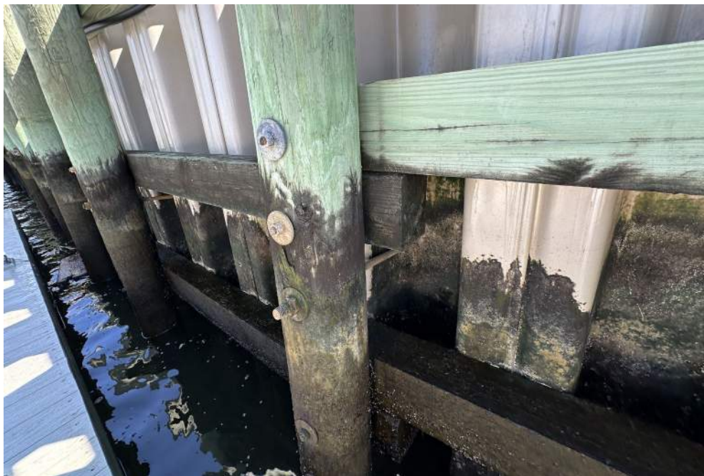
Photo 5: Section A, Easternly Bulkhead Waler Lap Connection, View 1
