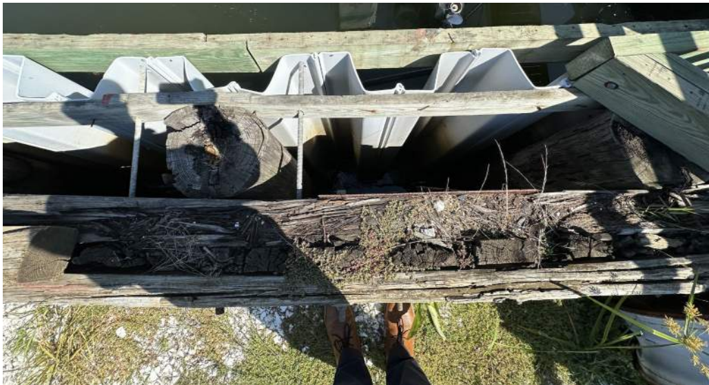
Photo 12: Section B , Southernly Bulkhead, Viewed Downwards from Grade
