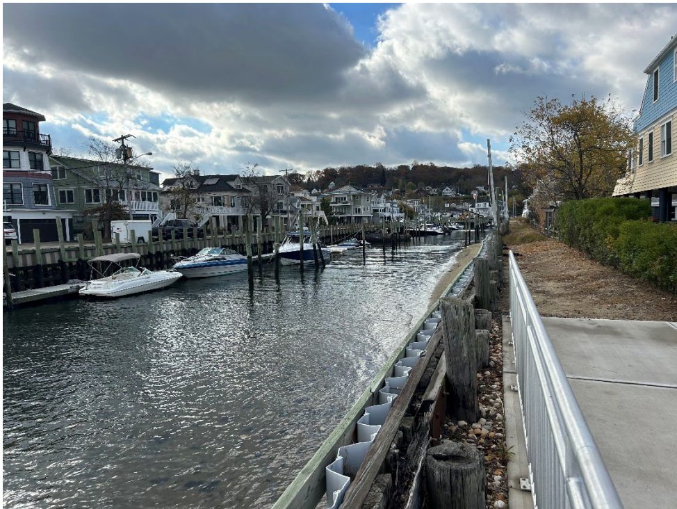
View looking down the Rogers Avenue Right-of-Way (11-11-2024) (Provided by HGA)
