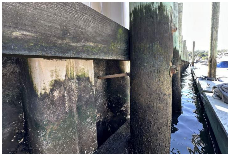
Photo 3: Section A , Eastern Bulkhead Exposed Fastening System View 1
