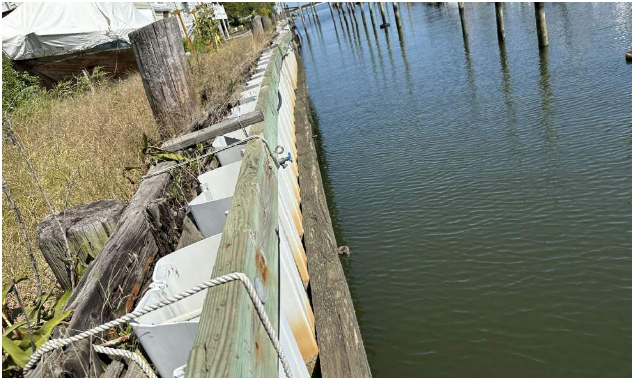
Photo 30: Section C , Westerly Bulkhead, Single Waler on Vinyl Sheet Pile, View 2
