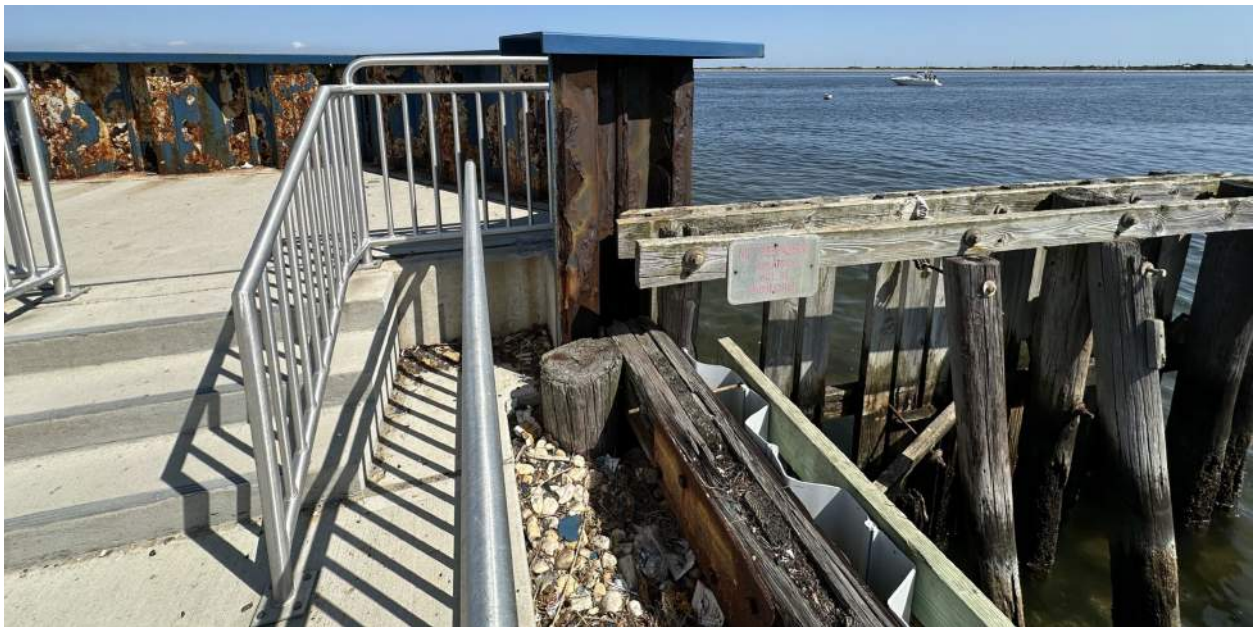
Photo 39: Section C, Westerly Bulkhead, Bulkhead Connection to Marine PI Bulkhead
