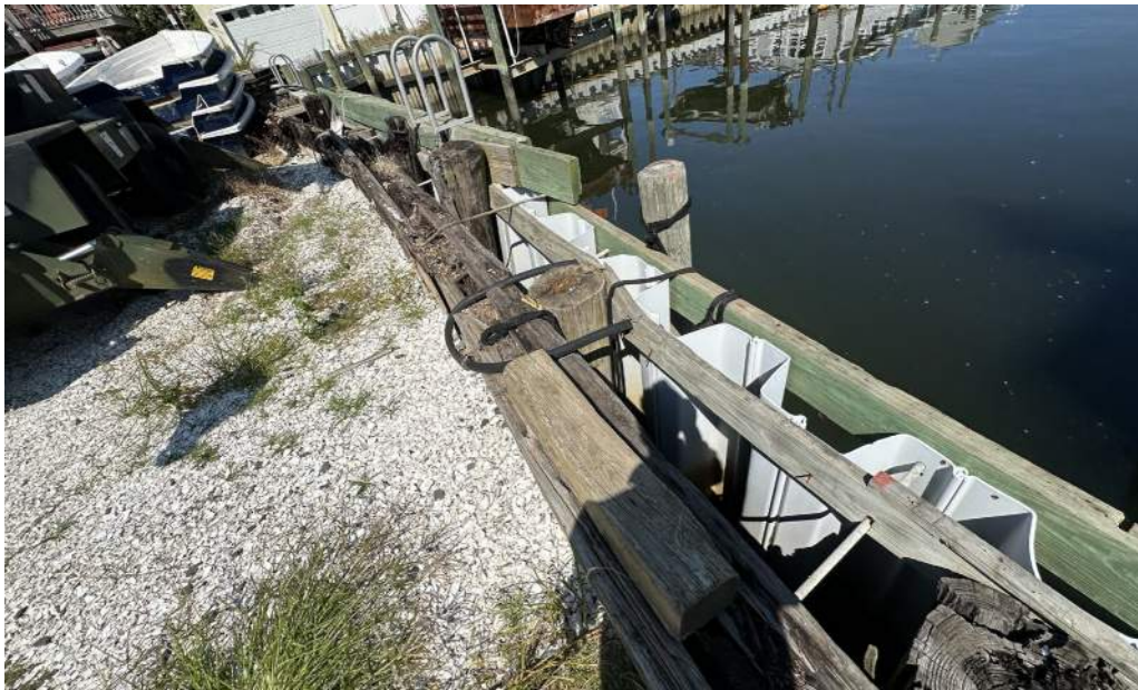
Photo 14: Section B , Southernly Bulkhead, Viewed on Angle from Grade, View 2
