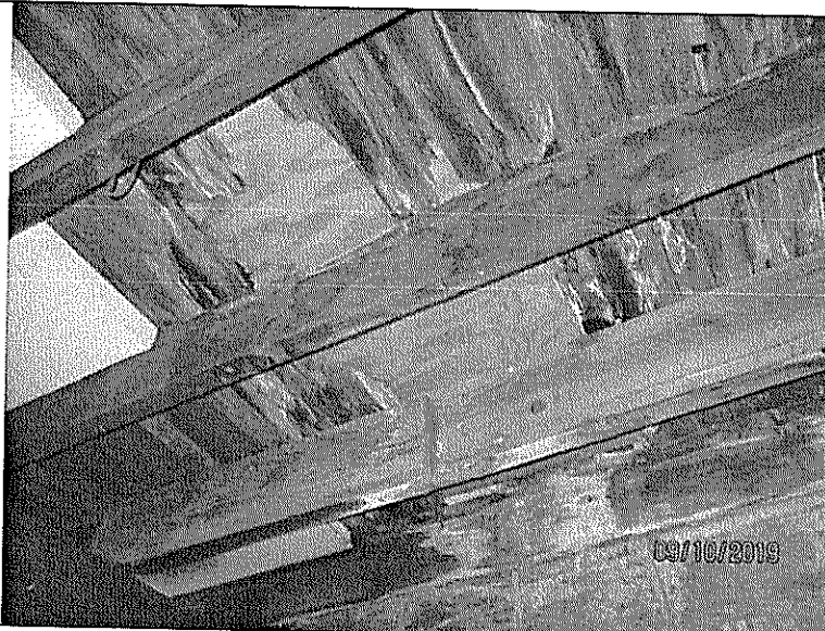
Photo No.: 8 (looking upward) Description: View of underside of second floor joists and flooring as seen from the first floor.
