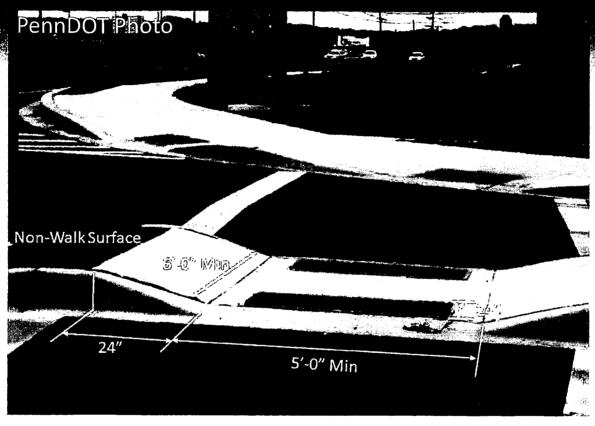
NJDOT Pedestrian Compatible Planning and Design Guidelines state if a street is wider than 60 feet than a pedestrian refuge should be provided so that people can find openings in traffic from only one direction, and have a place to wait for an opening in the other direction.
